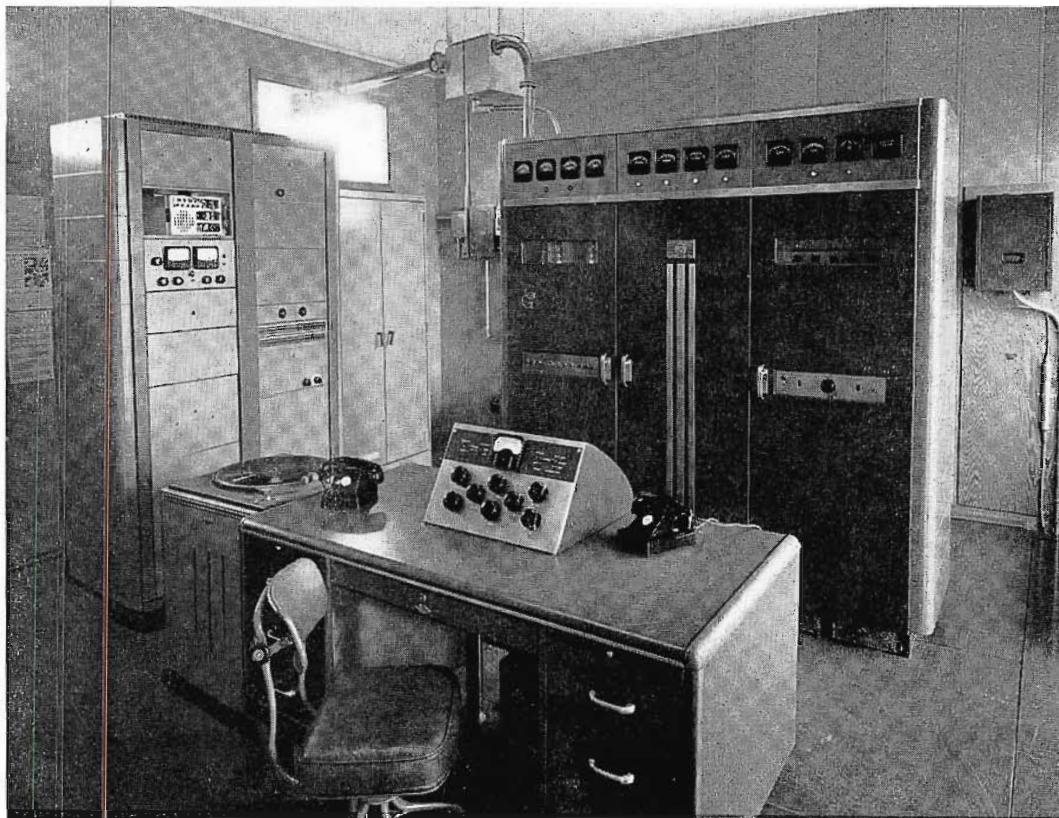
FIG. 11. View of the KOZY 3-KW FM Transmitter, RCA BTF-3B and Associated Console and Monitoring Racks.
