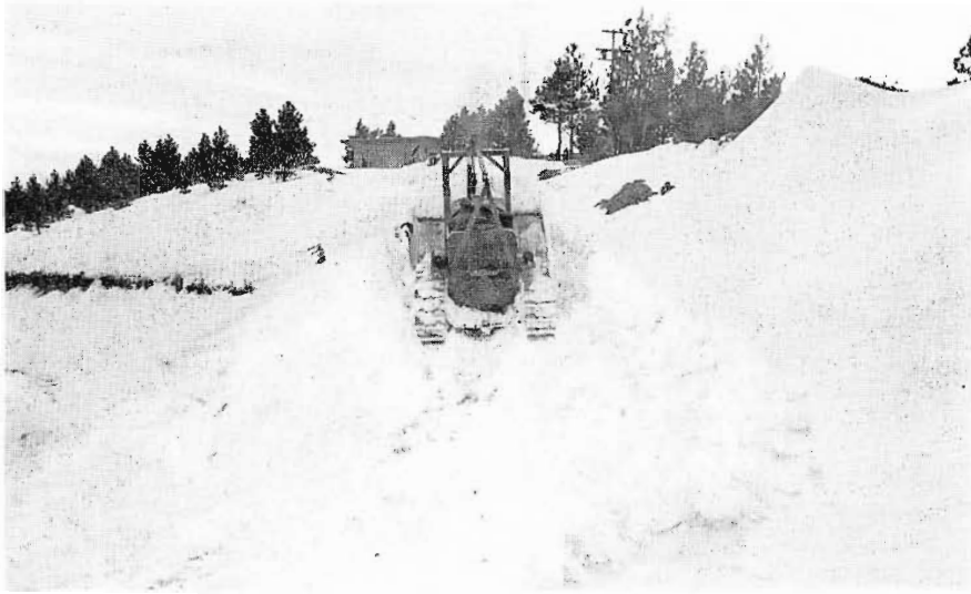
FIG. 8. View of a tractor opening the road to KOZY-FM plant atop "Signal Hill".
