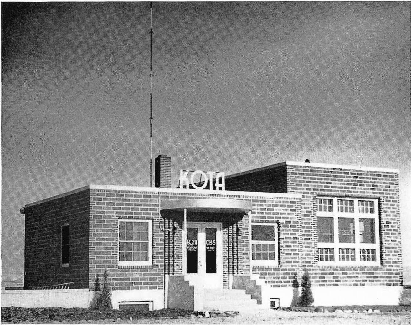
FIG. 4. Full view of the brick-constructed KOTA-AM transmitter building — located outside Rapid City.
