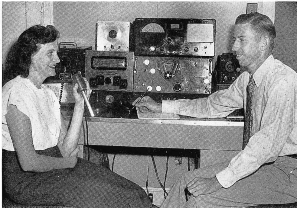
ABOVE are Inez and Bob Gordon in their ham shack, which is located in the WTJS transmitter building. Their 700-watt ham transmitter (not shown) is built into a 48-inch cabinet. Below, Inez is tuning up the exciter of the station's RCA FM transmitter.
